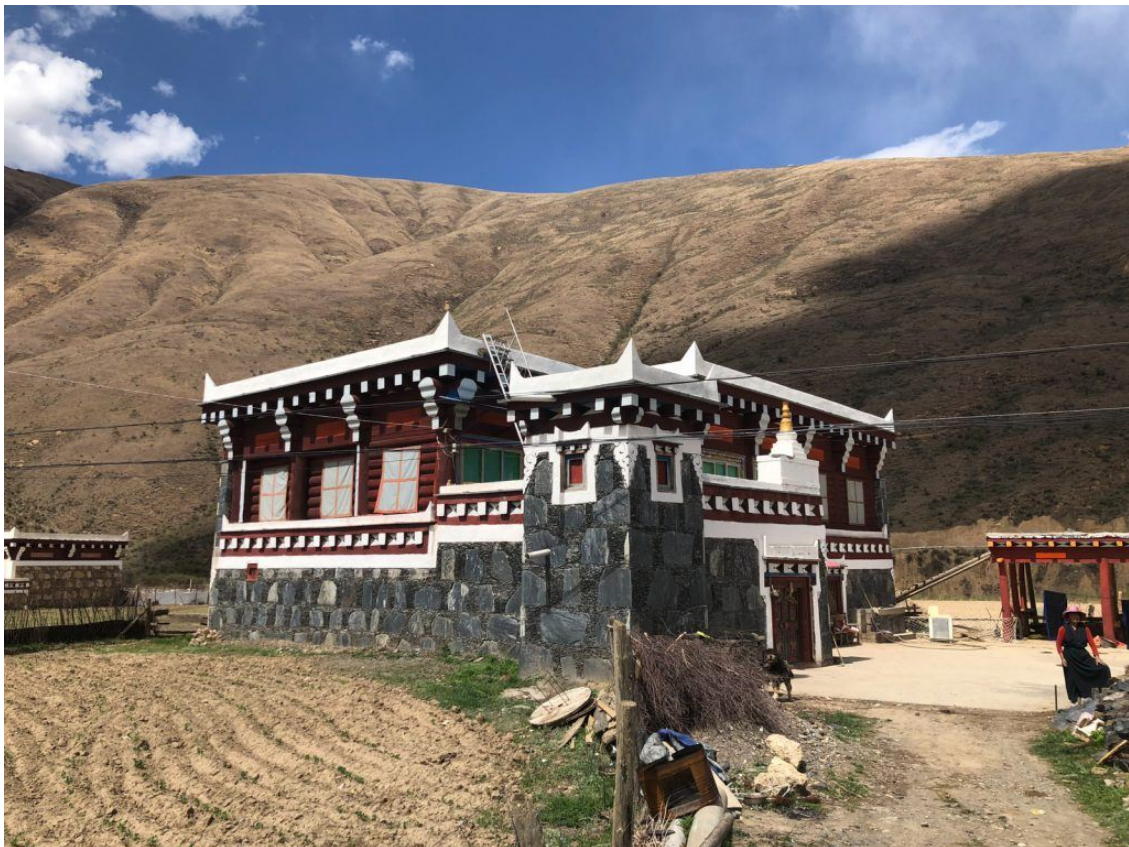
A Daofu traditional house in the village of Deerwa (Image by Inger Vandyke)
