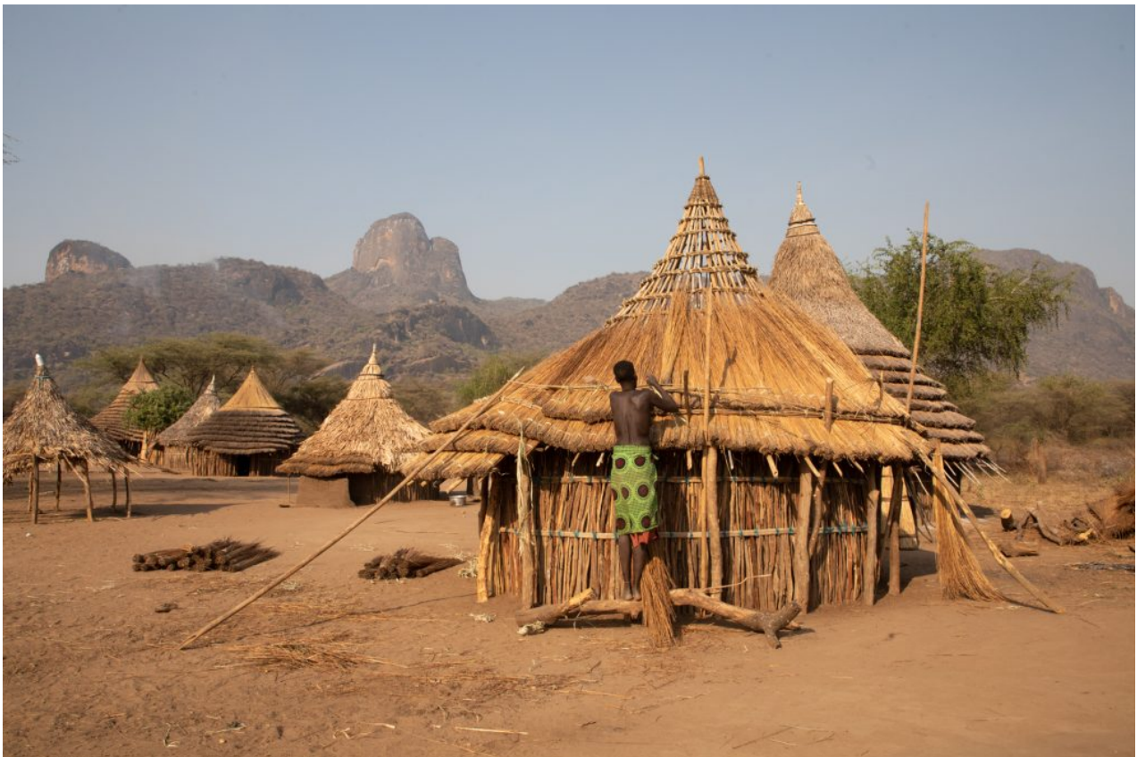
A Laarim woman stitches thatch to a new house being built in her village (image by Inger Vandyke)
