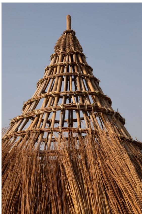
The internal structure of a Laarim hut roof (image by Inger Vandyke)
