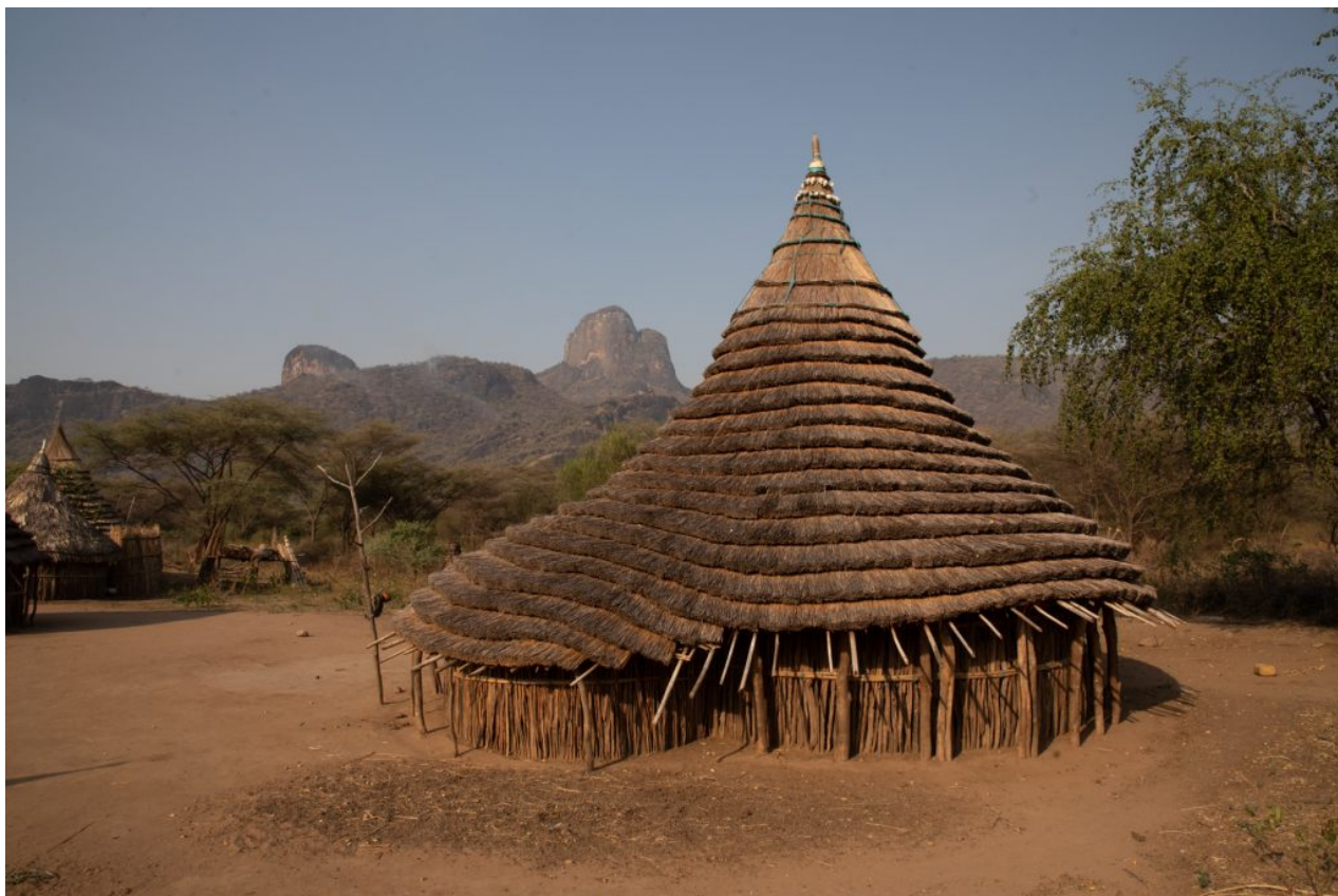
Laarim huts are a stunning example of African vernacular architecture (image by Inger Vandyke)
