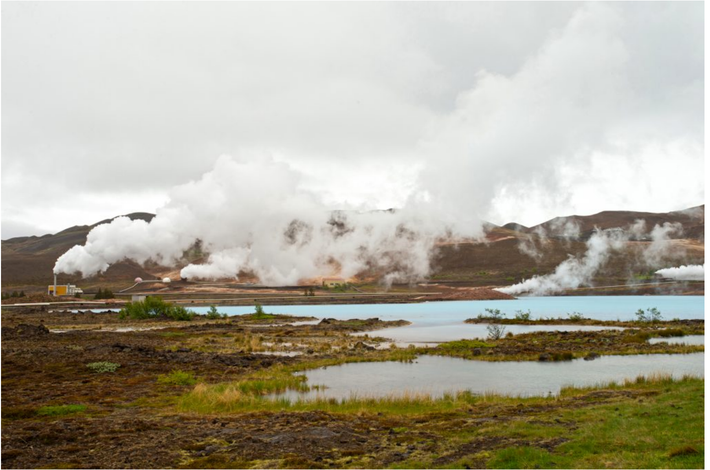
Geothermal energy plant at Lake Myvatn – Icelanders don't rely as much on gas and electricity for power as some! (image by Mike Watson)
