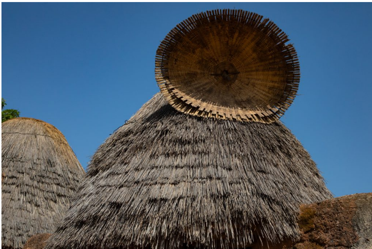
Each Otamari granary is split into four to store different items and all of them have a woven 'cap' to protect the contents from rain (image by Inger Vandyke)
